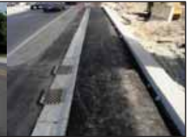
Richmond Canada Raised Bike Lane
